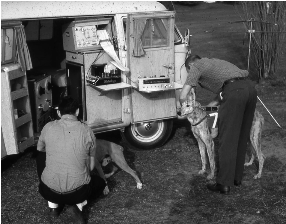
Fig. 8. Telemetry studies using a Volkswagen bus equipped with standard consumer high-fidelity audio equipment to record Doppler flow signals from instrumented dogs.
